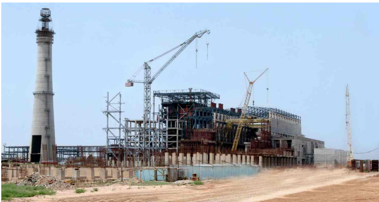
Rehabilitation of a power station
