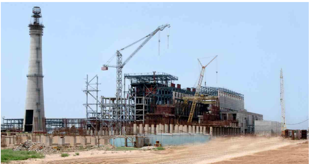
Rehabilitation of a power station
