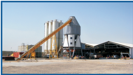
Abu Ghraib Concrete Sleeper Factory
